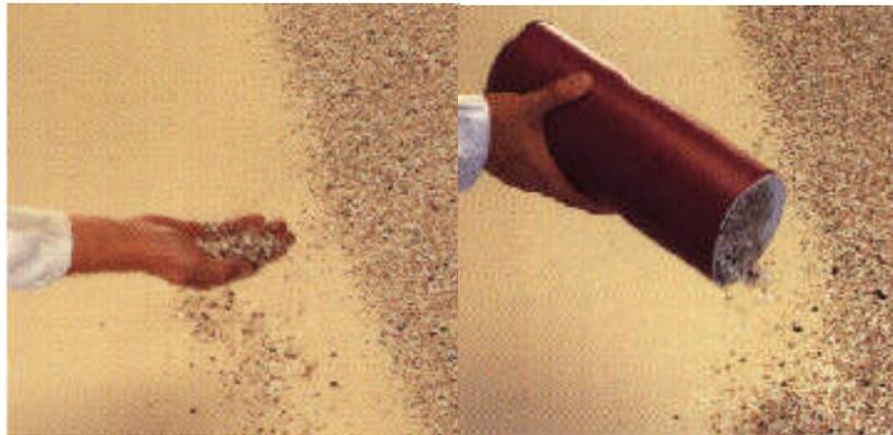
**Step 3:** The transparent top coat, which is applied in one or more layers. As dazzling as the visual effect is, there is more to making a product successful. There are many factors contributing to the success of Epoxy Systems' Flake Flooring.
