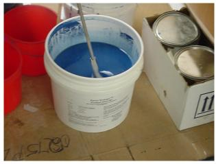
Stir the Resin "A" and the Hardener "B" each separately in there original container before measuring and mixing the two together. Be careful to use separate stir sticks so not to cross contaminate.
